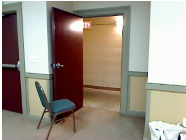
Typical Work Area Four Required
