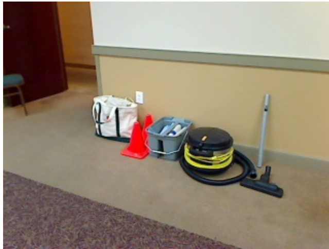
Typical Renovator Work Supplies
